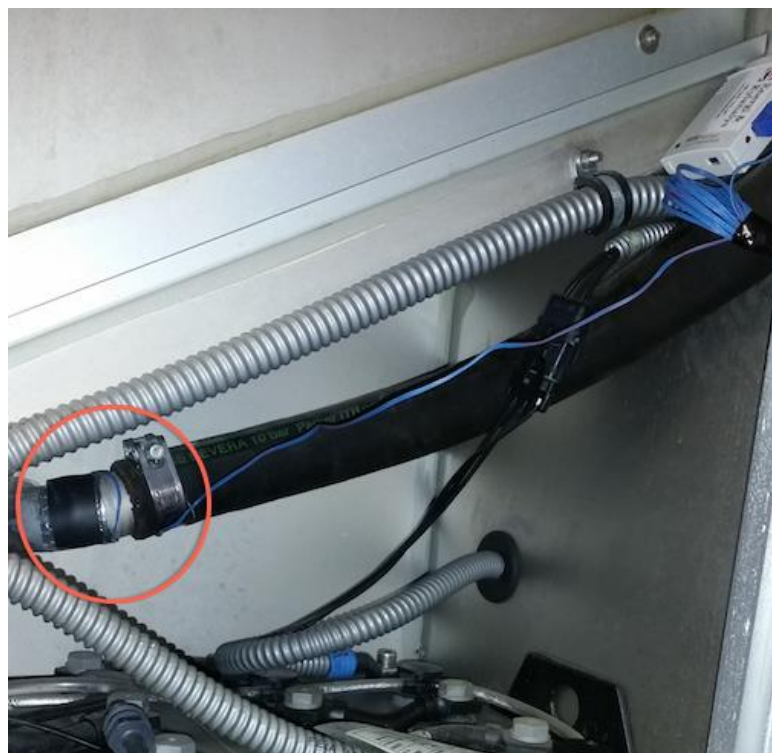
Figure 51. Temperature logger attached to resurfacing machine water inlet
