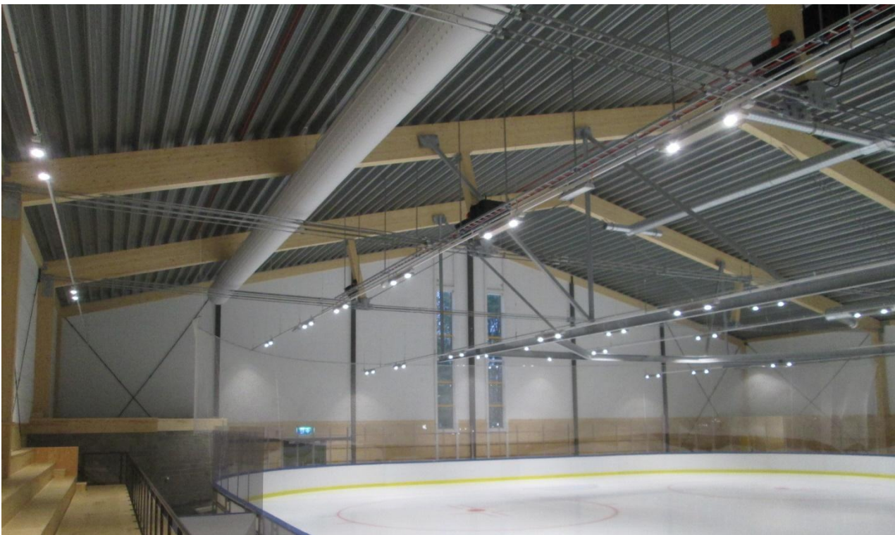
Figure 1. A newly built ice rink with large elements of wood and perforated sheet metal in the walls.
