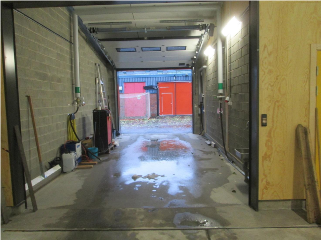
Figure 12. Example of an ice machine garage with roller doors at both ends, both of which are open!
