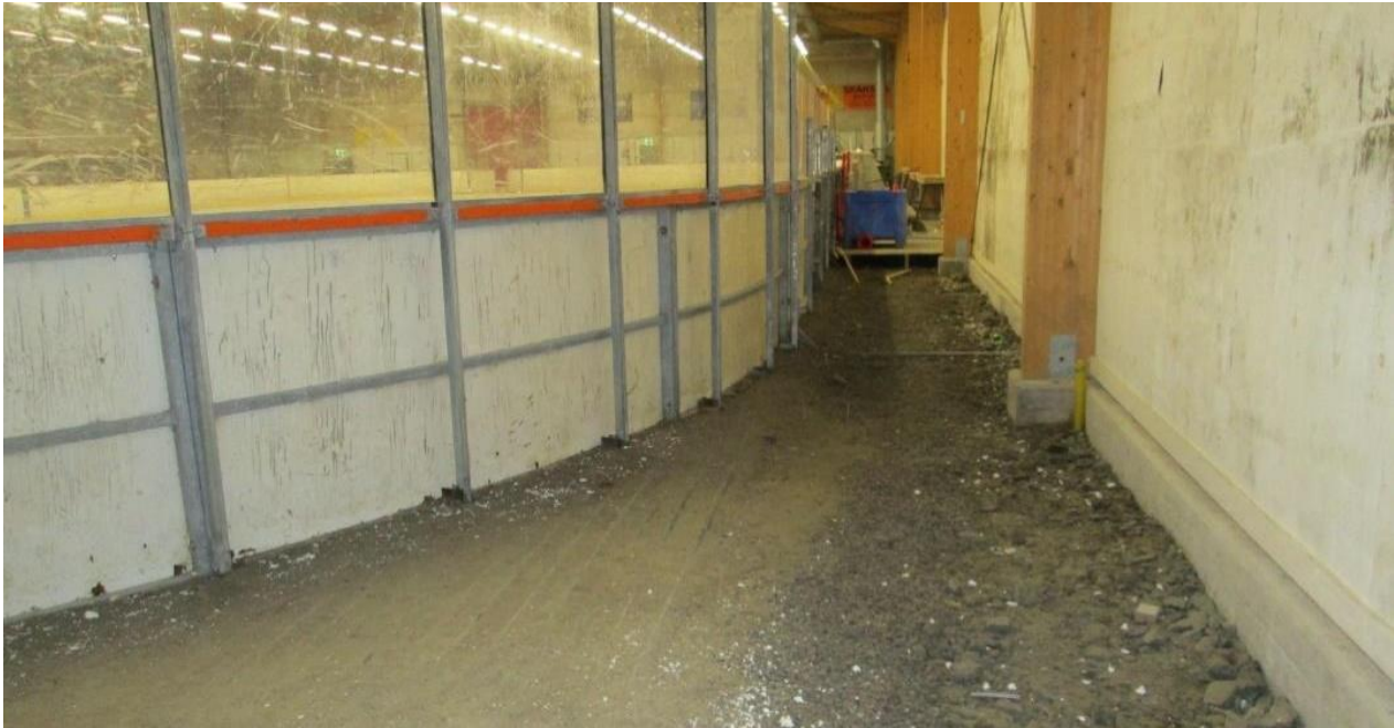
Figure 9. Gravel rink where even the surrounding surfaces in the ice rink are completely or partially "open", i.e. they have no covering layer.
