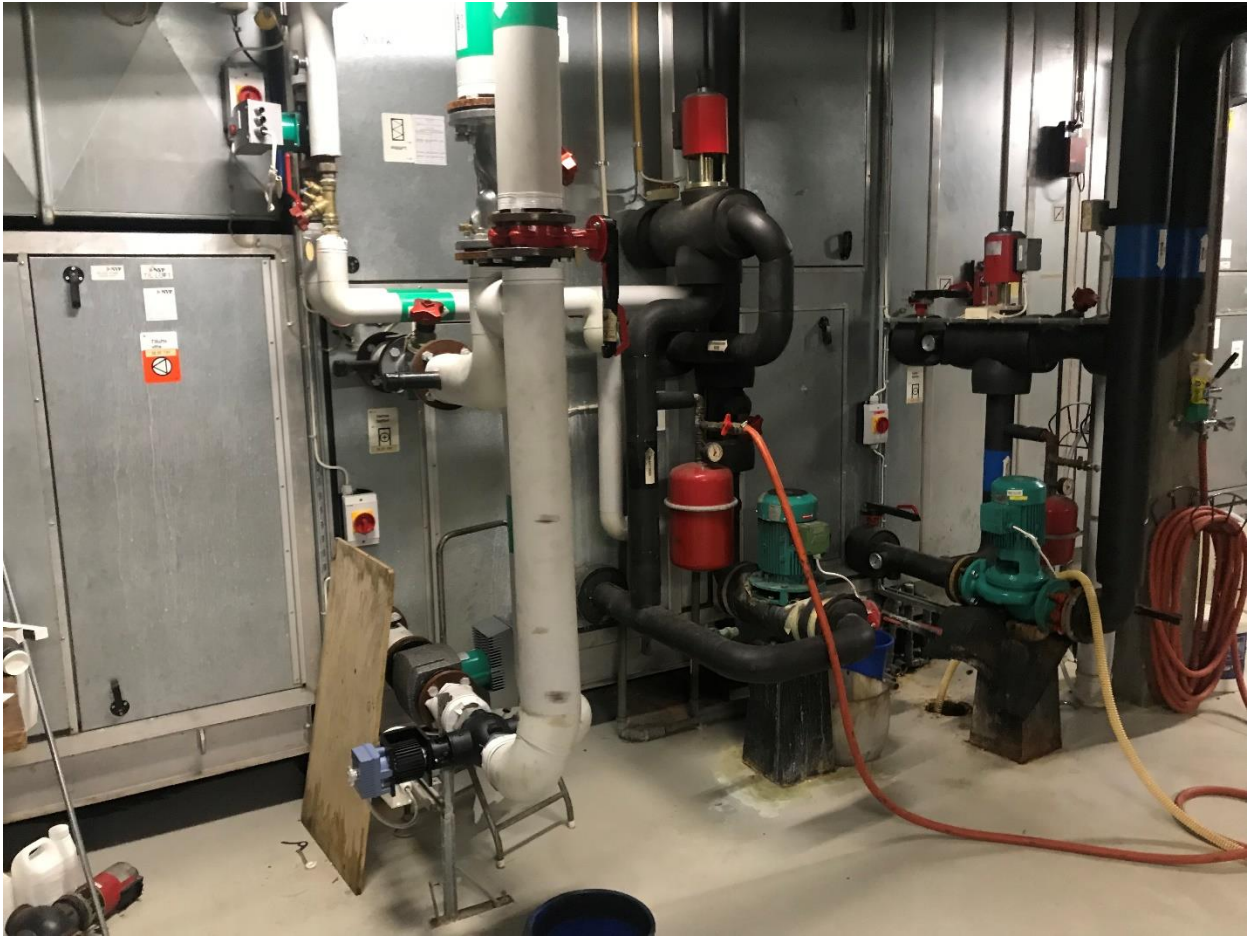
Figure 4. A ventilation unit with an indirect refrigeration dehumidification function.
