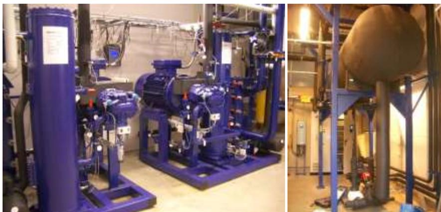
Figure 6. The Backavallen ice rink in Sweden with CO<sub>2</sub> as secondary refrigerant in copper tubes.
